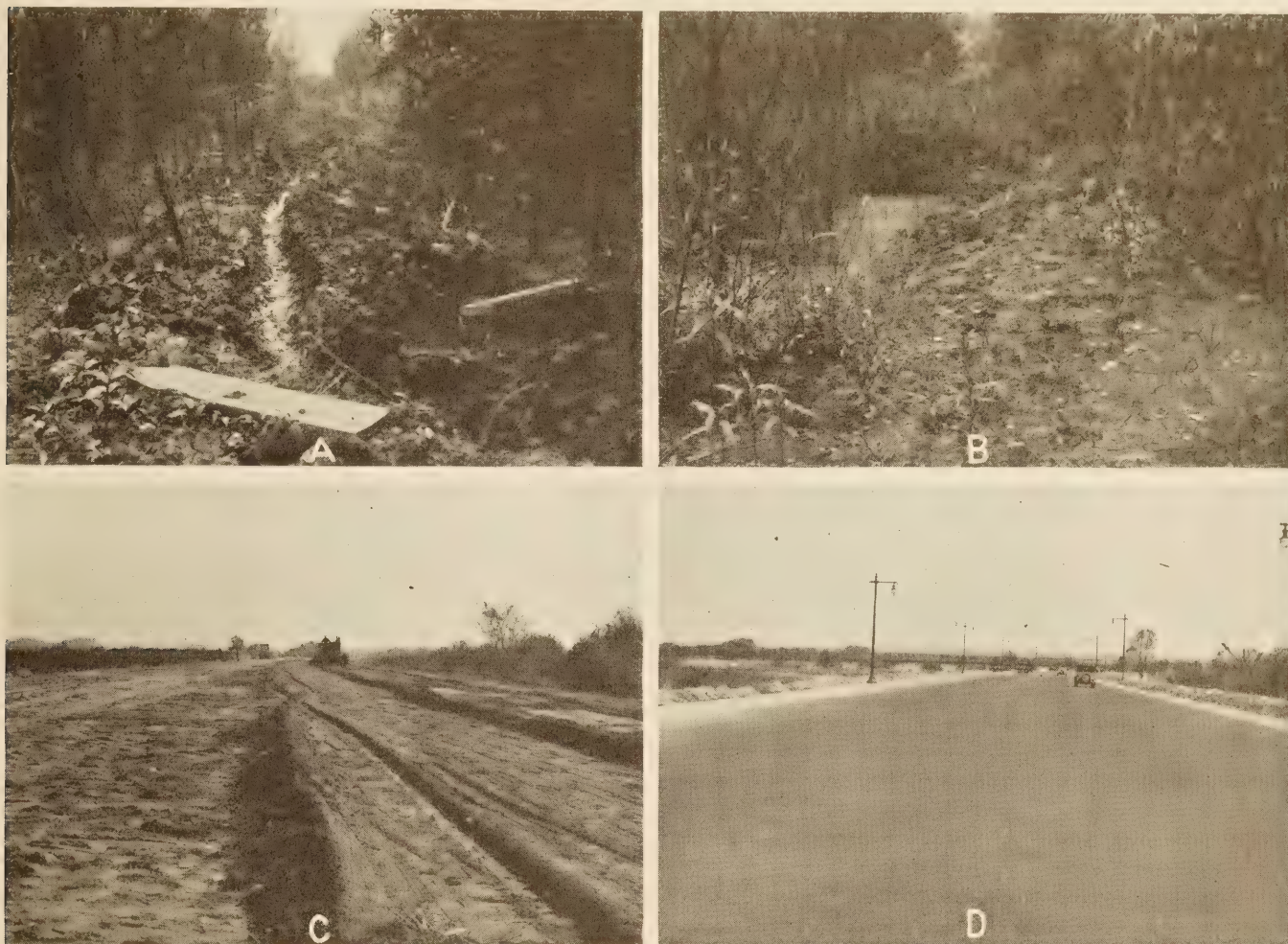
FIGURE 8.—PHOTOGRAPHS TAKEN AT STATION 10+00, AT DIFFERENT STAGES OF THE WORK
